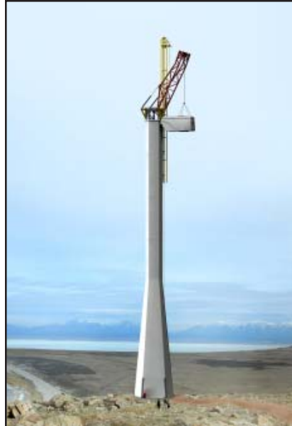
Fig. 4 - Lifting Nacelle
