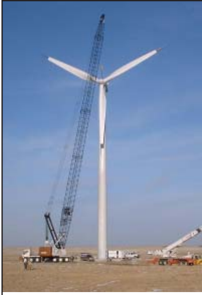
Fig. 1 - Heavy-lift crane installation
