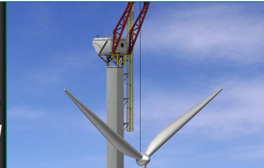
Figure 5. Space frame wind tower with Hi-Jack and gin pole
